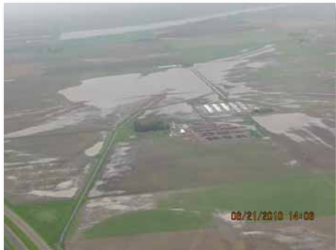
Figure 1 Flooding at the Confluence of the Malloy Drain East of the Town of Coaldale, June 21, 2010
