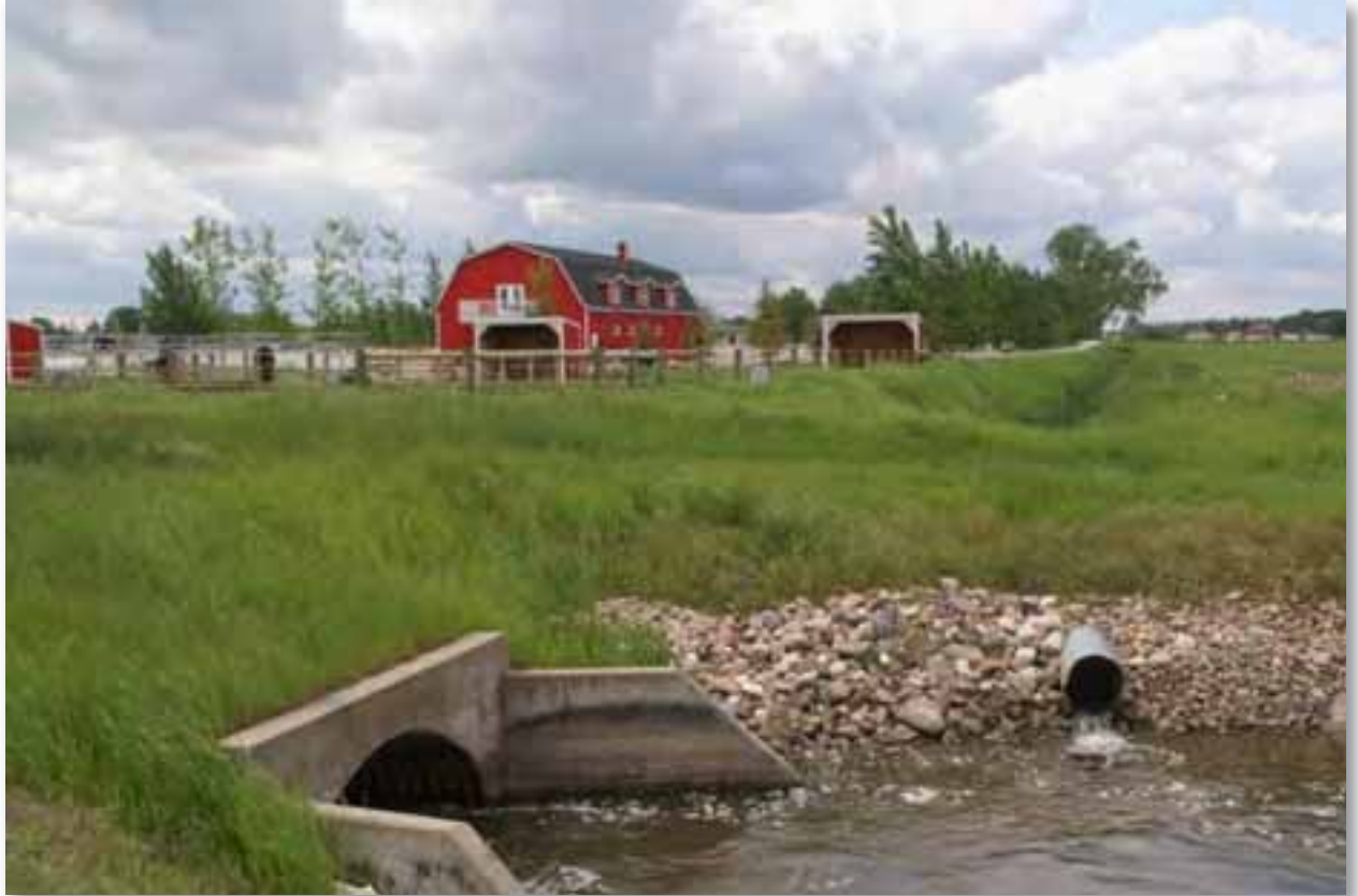
Point at which the Regional Pathway would turn West from the Canal to Follow Private Lands
