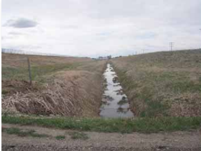
Figure 12 South Coaldale Lateral (right), Drain (centre) and Abandoned Raw Water Reservoirs (left), May 5, 2011
