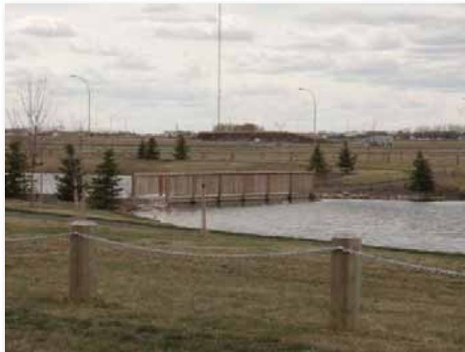
Figure 17 Stormwater Management Pond at Broxburn Business Park (May 5, 2011)
