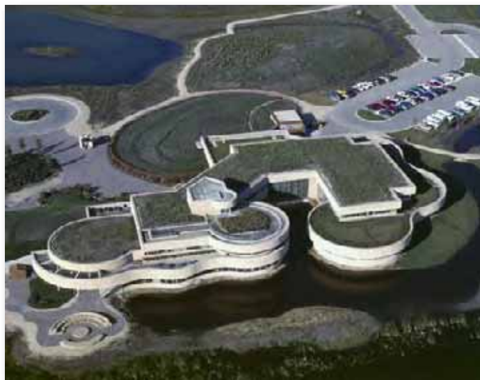
Figure 16 Green Roof on the Ducks Unlimited Headquarters in Winnipeg, Manitoba
