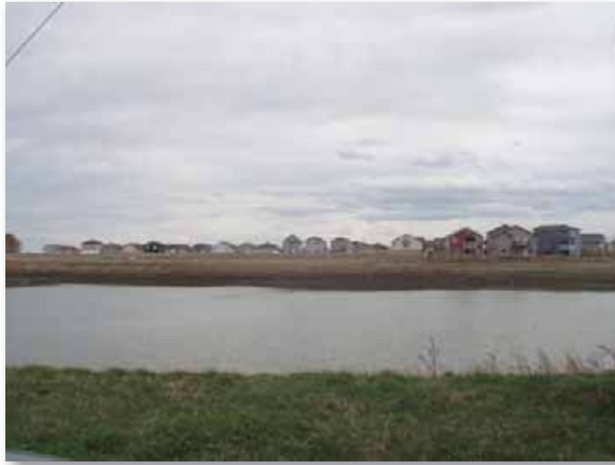
Figure 11 Main East Storm Pond within the Town of Coaldale, May 5, 2011
