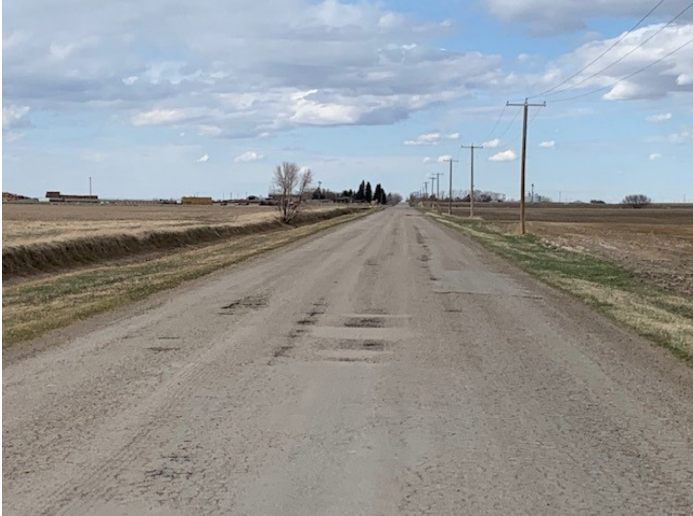
Picture 7: 1.5 miles north of Hwy 519, more alligator surfacing
