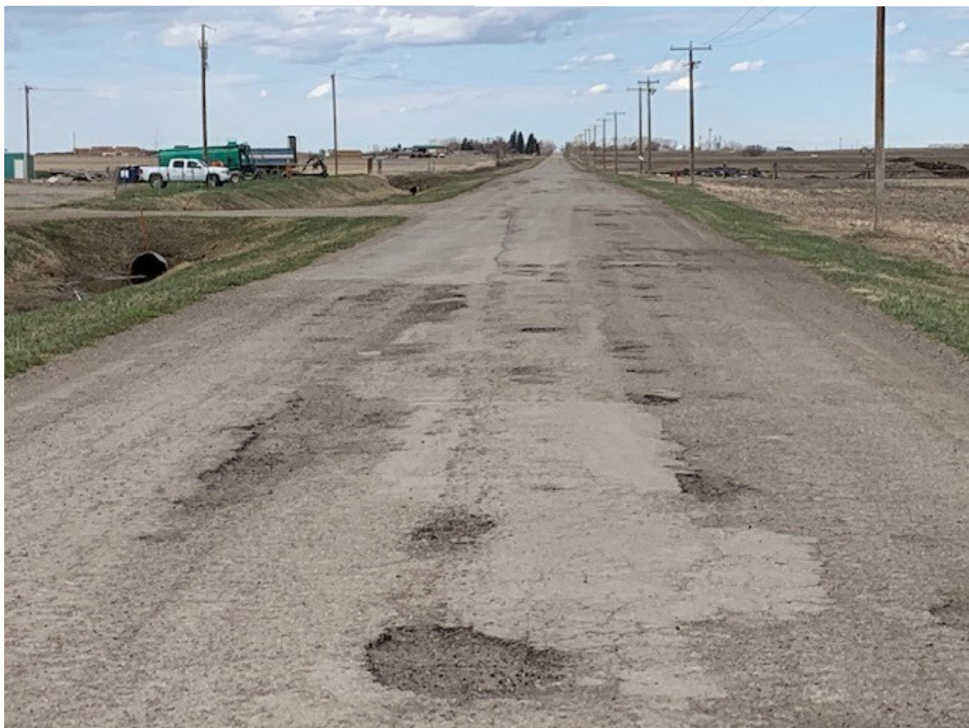
Picture 6: 1.5 miles north of Hwy 519, alligator road surface
