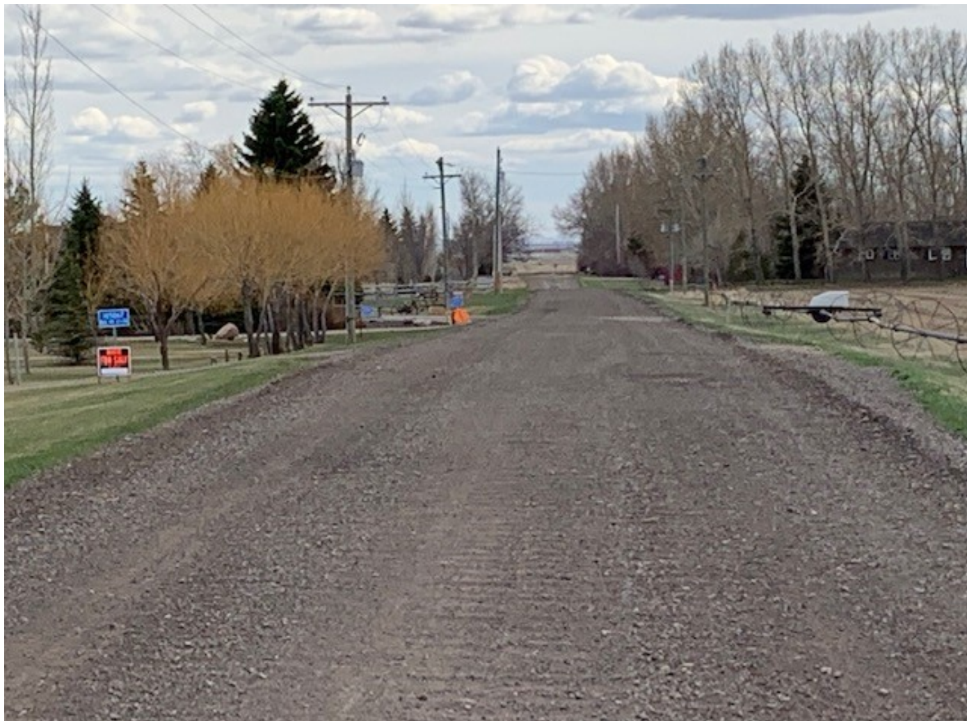
Picture 4: 400 meters south, Washboard from roughened surface
