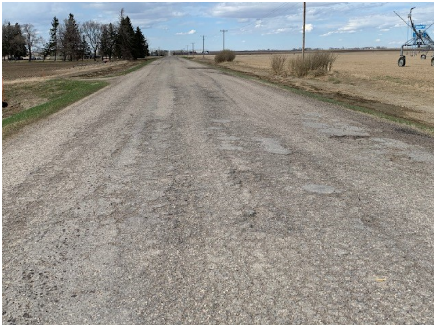
Picture 2: 300 meters north of Hwy 519, severe ravelling of road surface
