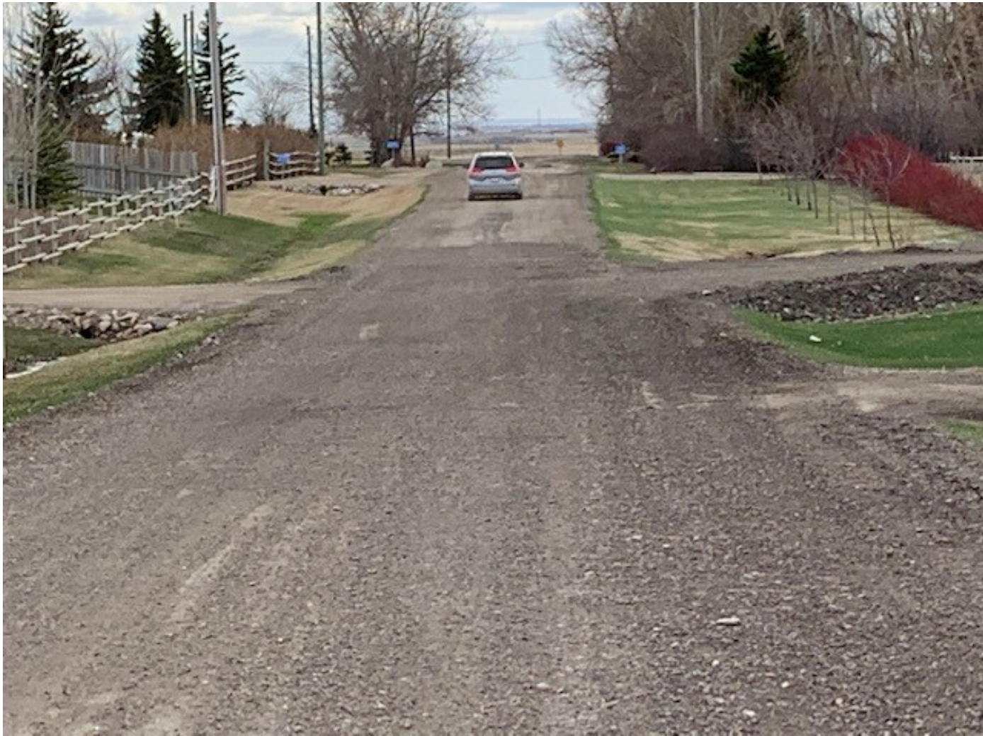
Picture 5: 800 meter south, Road is milled surface, no compaction
