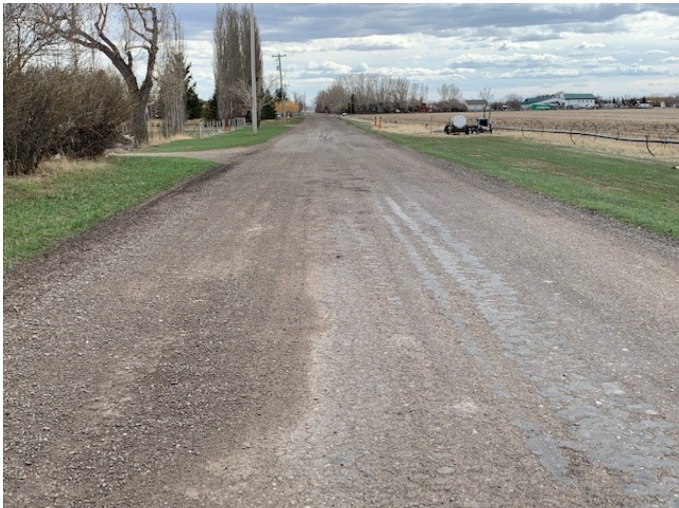
Picture 2: 100 meters South of Hwy 519, Road Surface Ravelling
