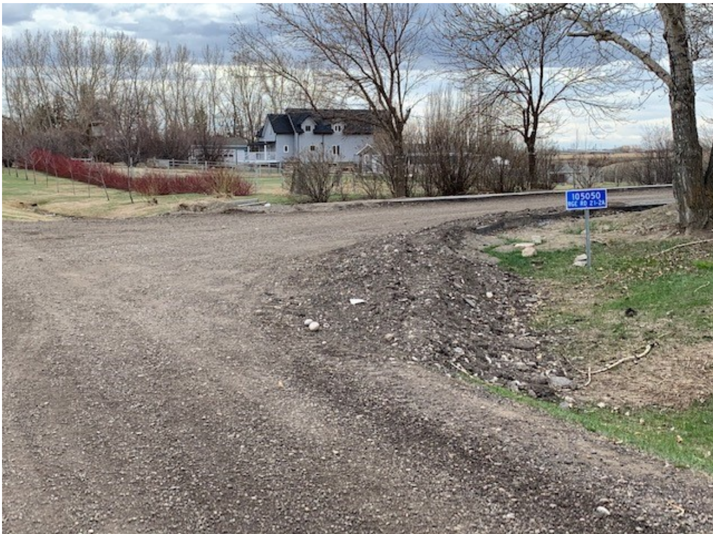
Picture 6: Landowner Entrance, road material rolled into ditch by unauthorized grader
